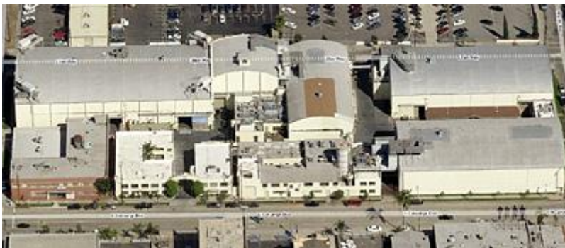
aerial view of Red Studios
