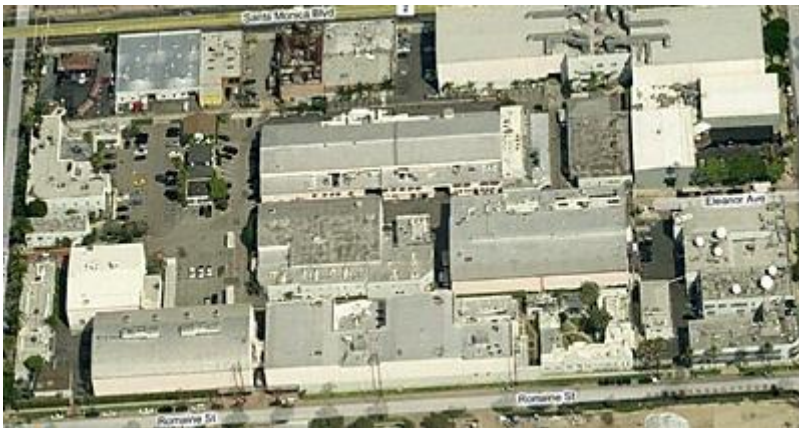
aerial view of Hollywood Center Studios
