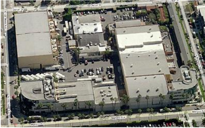
aerial view of Raleigh Studios (Bing Maps)
